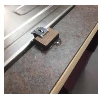
**Top Tip:** Support your Evolve worktop as you work through each process particularly at the point of creating the sink cut-out as this could lead to a temporary weakening of the worktop.
