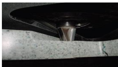
(4) Rout bevel into counter
