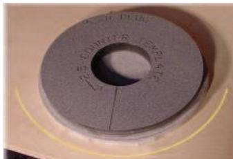
(5) Cut repair piece 9.5mm( \frac{3}{8} ") bigger than template Hot melt together
