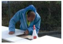
When sanding the inner corners it may be necessary to peel off the velcro backer from the diamond sanding pads to improve flexibility for accessibility.
