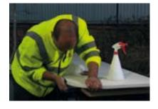
When using sanding pads ensure both the M-Stone edge and the sanding pad are kept moist; use a hand held spray bottle filled with pure water.
