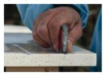
During hand sanding keep the drainer groove and the radiussed sanding pad moist by spraying with pure water.
