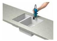
Try to trim back in several light passes to minimise cutter/bearing wear. We recommend extraction to reduce dust.
