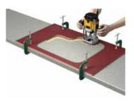
Using a 30mm guide bush and 1/2 inch router cutter, form a full depth cut-out, ensuring the waste section is supported to prevent damage as it falls away. Router cut in stages at 15mm depth.
