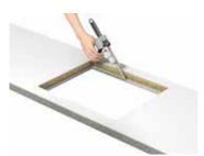
Apply two unbroken 4mm beads of Encore colour coded seaming adhesive to the inner corner of the cut-out and approximately 4mm in from the cut-out edge on the solid surface.
