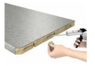
Apply two 5mm beads of adhesive along the entire length of the joint.
